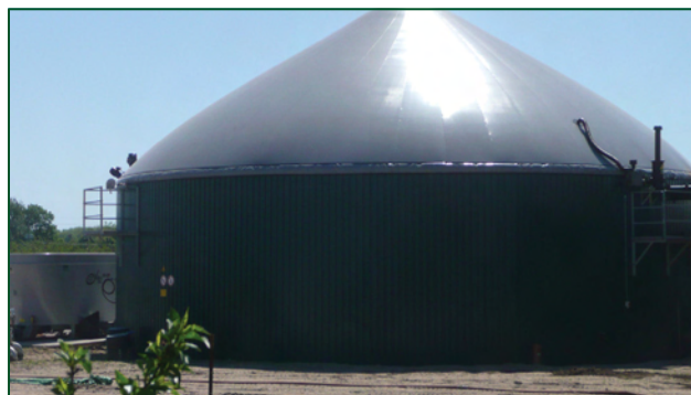
Anaerobic digestion facility
